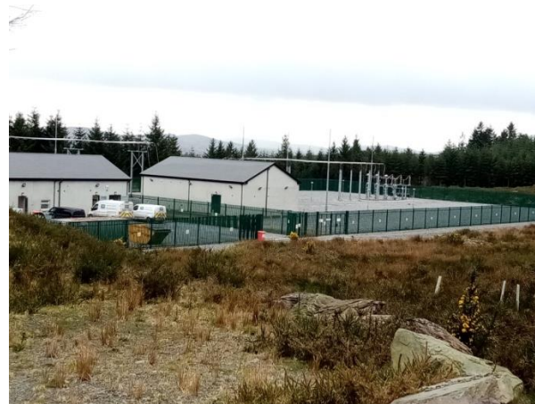
Carrigerierk wind farm. Examples of the amount of infrastructure required.
